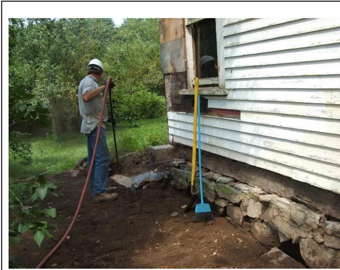
**Figure 58 Foundation Cleaning**
