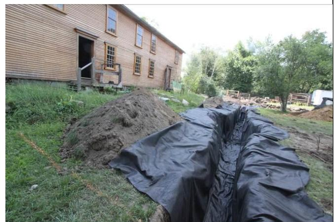
**Figure 113 Drainage in Rear of House**
