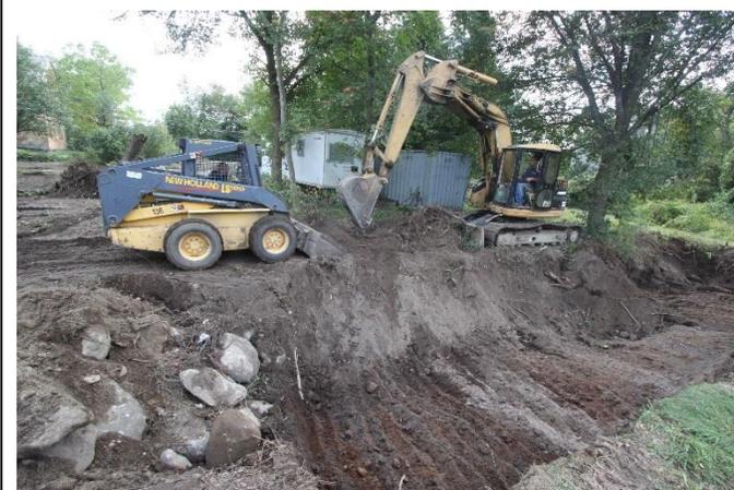
**Figure 114 Drainage Ditch to Rear of Barn**
