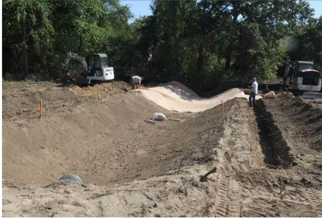
**Figure 116 Drain Outlet Ditch During Construction**
