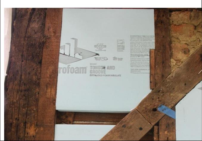
**Figure 27 Insulation Added When Possible**
