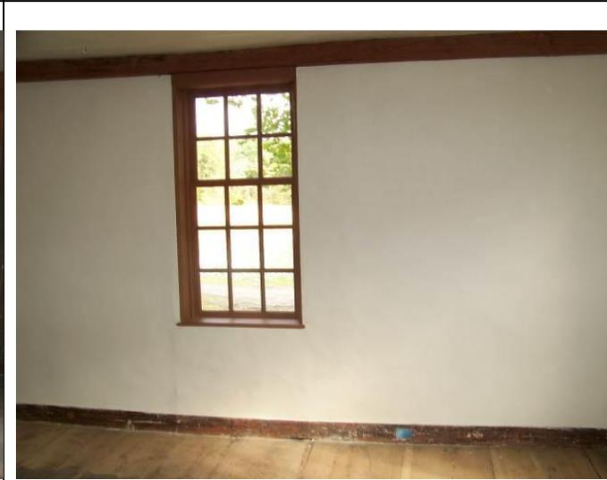
**Figure 47 Wall with finish coat**
